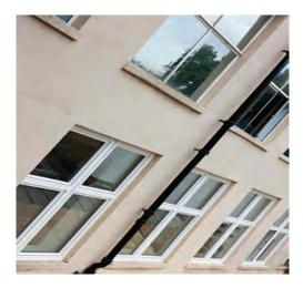
On the first floor of The London Building Centre in Store Street, seven tilt and turn GENEO<sup>®</sup> windows have been installed to replace 1960s aluminium frames as part of an overall refurbishment programme which is aiming to achieve a BREEAM Excellent rating.
